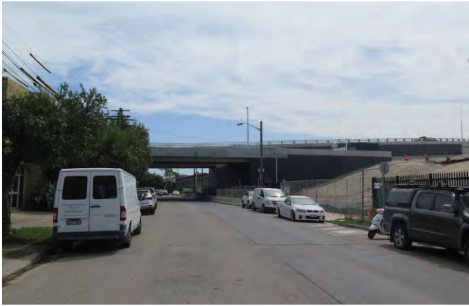
View 5 Existing - View from Burrows Road, looking South-West towards site
